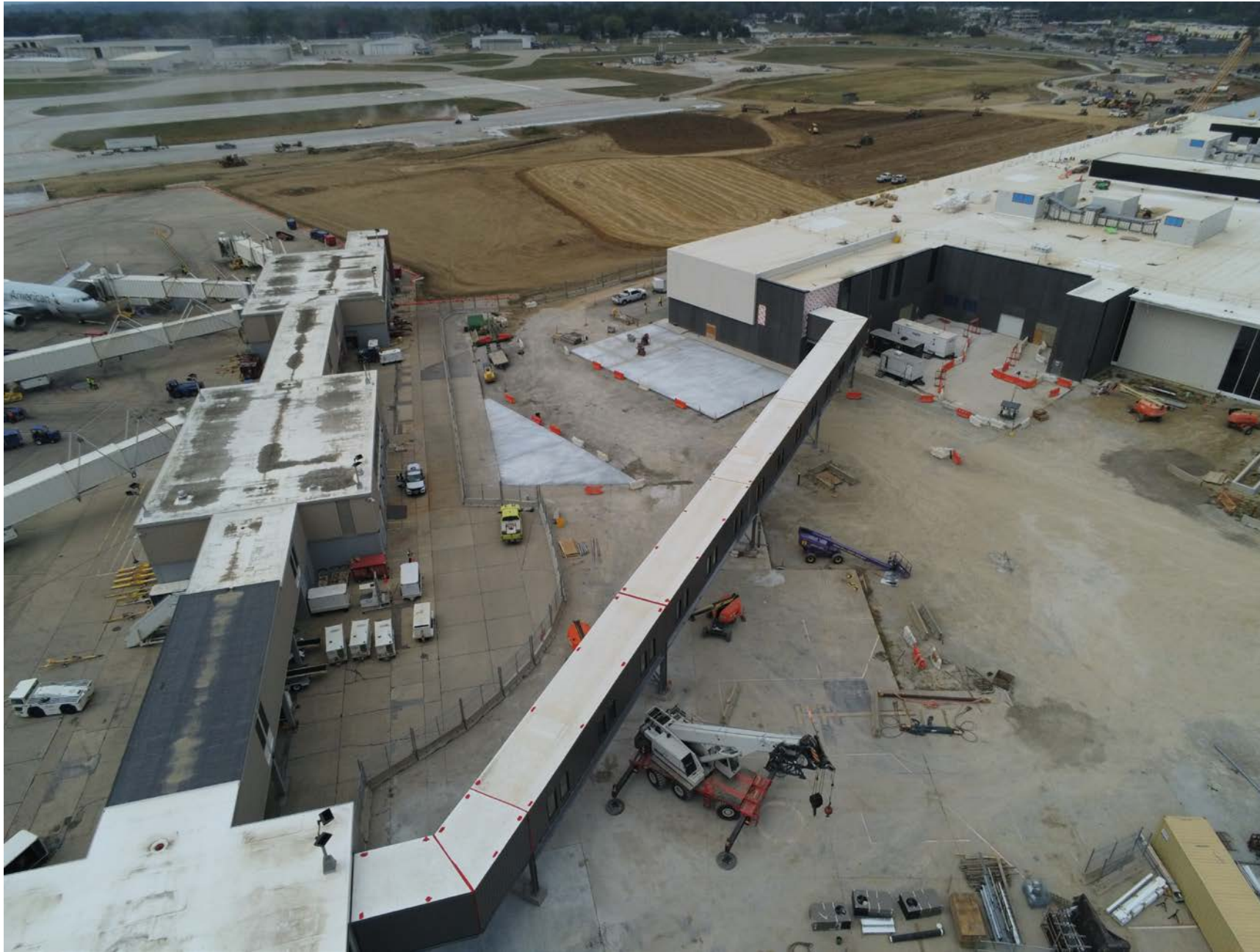
Skyview of the passenger walkway connecting the New Terminal to the existing Concourses
