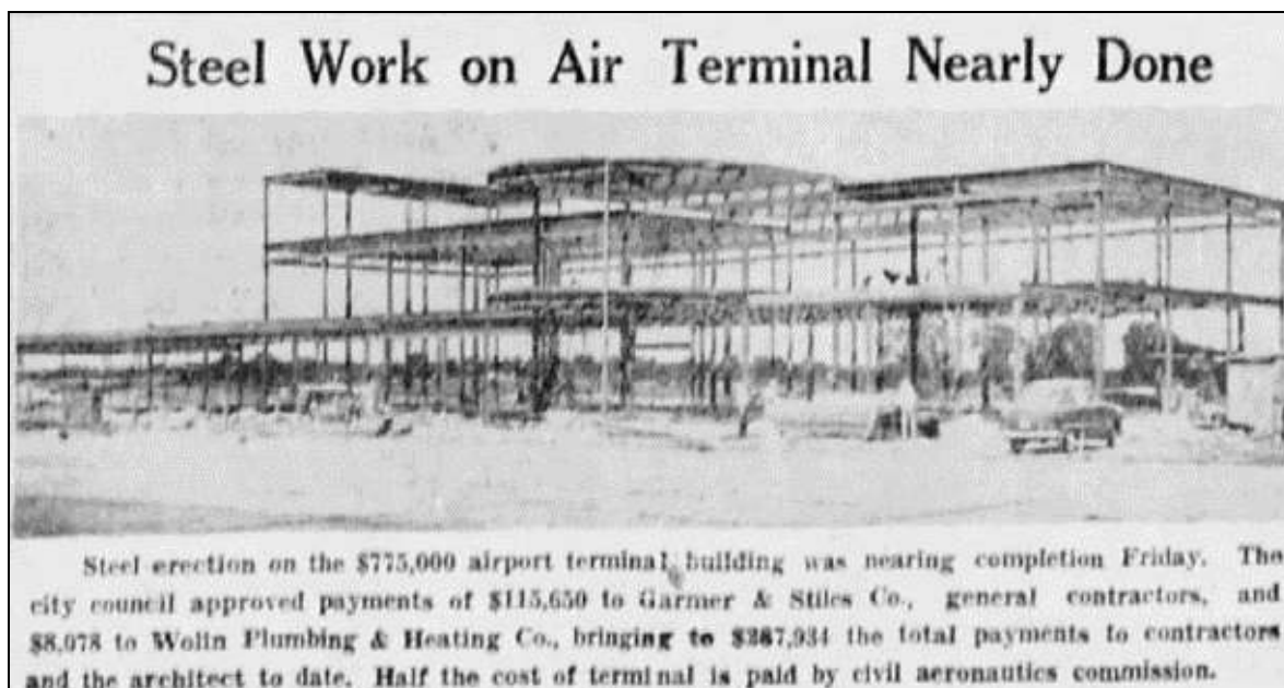
Figure 10. Image from the Des Moines Register of the steel frame work of the new terminal building under construction. (Source: Des Moines Register , 8/13/1949).
