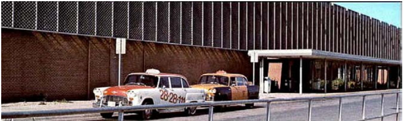
Figure 24. 1960s postcard view of the remodeled east front (looking northwest) of the expanded terminal before the larger, full-length, sidewalk canopy was added. Ground floor windows have been bricked in and a metal screening added to the second level (nonextant). (Image obtained from the Airport collection).
